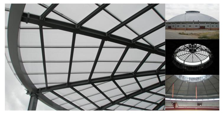
The structure for the bullring roof in Arroyo de la Encomienda is conceived as a laminated structure with a dome-shaped form having a 53.90m radius set upon a circular 34.45m radius plan giving a rise/span ratio of 1/5.3.
